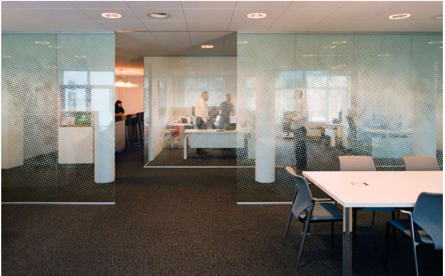
OFFICES WITH GLASS SCREENS, COVERED WITH AN ABSTRACT, SEMI-TRANSPARENT PRINT
